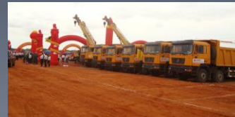
Building social housing in Angola
